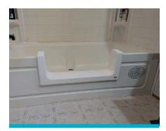
Pictured here is an example of a successful "tub cut" bath modification.
