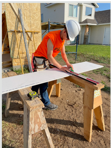
Photo: Michael working on a Habitat for Humanity project.
