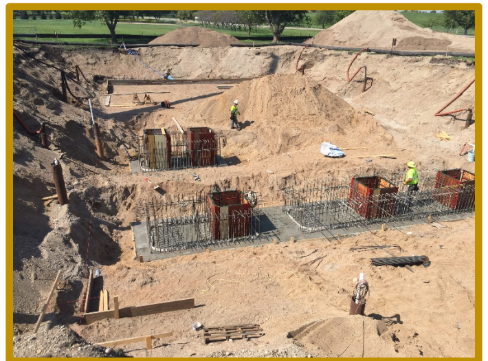
Early construction of the Morris Water Treatment Plant
