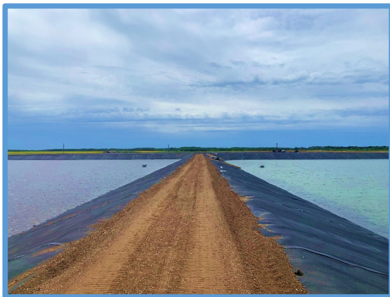
Wheeler's Point Sanitary District wastewater collection and treatment system
