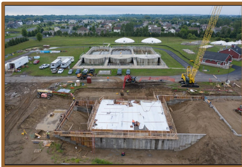
City of Otsego Construction of the Biosolids Processing Building
